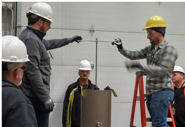
Left, Hopewell Designs employees remove the lid of a shielded containment vessel holding an 830-curie Cesium-137 source, while DOE-Idaho RESL and BEA personnel monitor the work.
